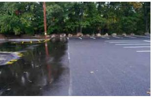
Traditional asphalt on left, permeable on right.
